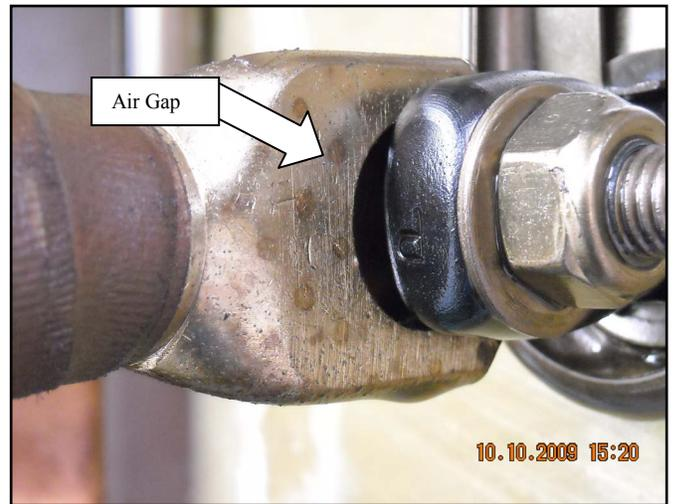
Figure 10: Cable Lug with Gap (T6, T10, T11, T7)
